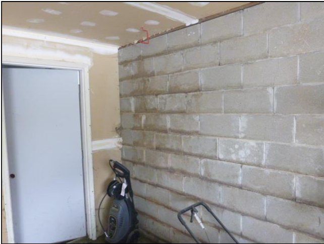
4.0 Item 1(Picture) area behind exterior stoop
