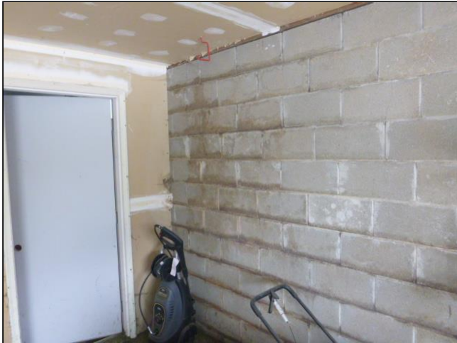
4.0 Item 1(Picture) area behind exterior stoop
